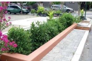
FIGURE 3. PHILADELPHIA WHERE RETROFITTING GREEN INFRASTRUCTURE TO MANAGE STORMWATER IS DE RIGEUR (COURTESY M MAIMONE, CDM SMITH)
